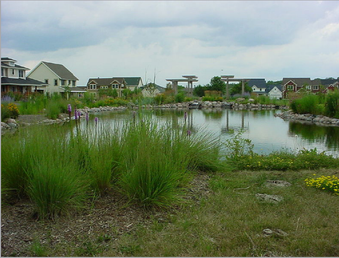
Figure 5: Retention pond in a subdivision (credit: Minnesota Stormwater Manual)
