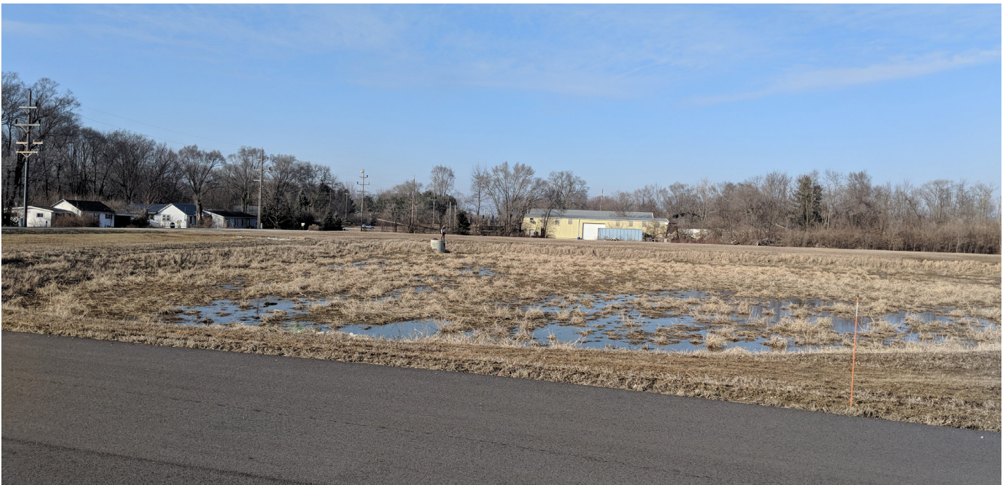
Figure 7: Detention basin draining runoff from a large parking lot
