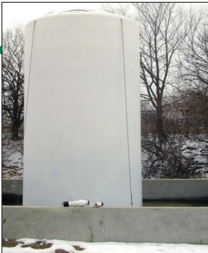
Vertical storage tanks should be secured. Notice the tie-downs on the tank shown in these two photos.
