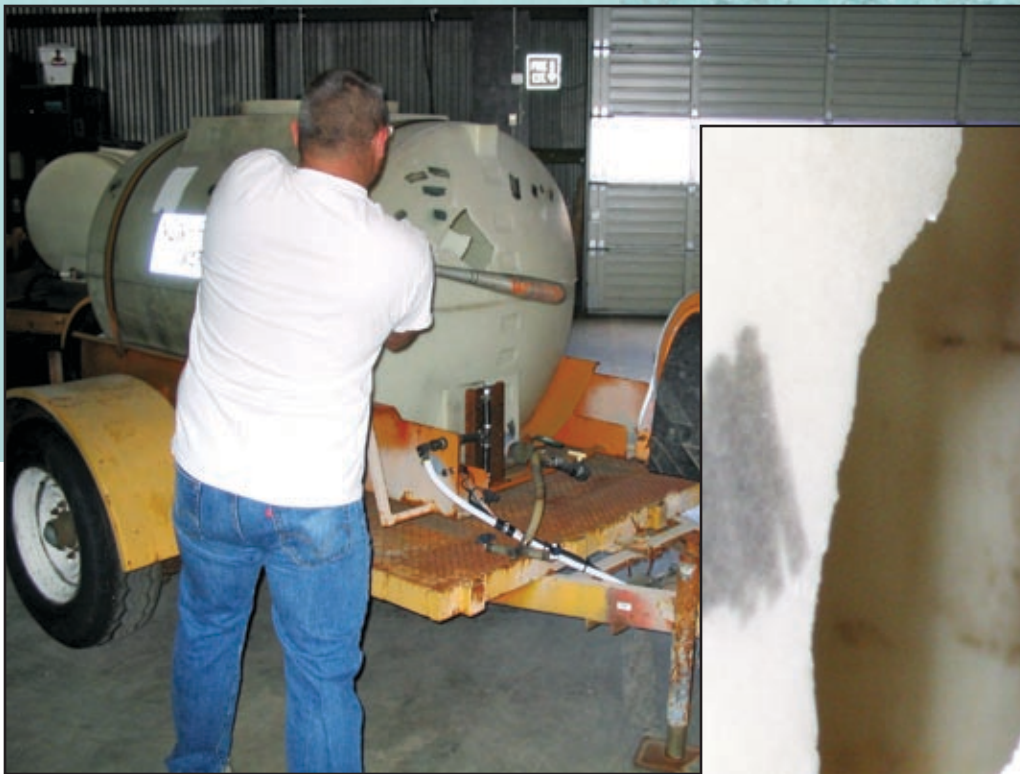
The tank above showed significant UV damage; and when tested using the ball bat method, it broke open. The plastic was brittle across the width of the tank (right).
