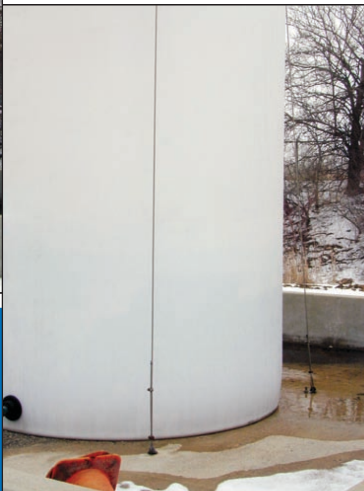
Vertical storage tanks should be secured. Notice the tie-downs on the tank shown in these two photos.
