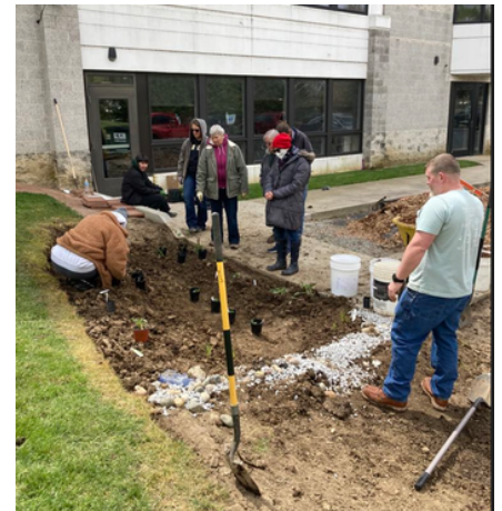
Rain garden at the library
