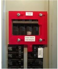
A two-pole 120/240V circuit breaker will need to be added and it should be placed according to the instructions of the interlocking kit. Other circuit breakers may need to be relocated.
