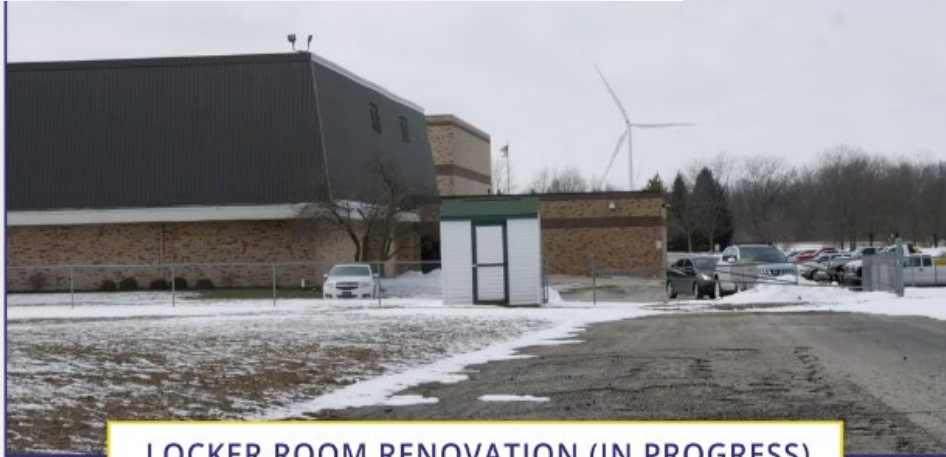
LOCKER ROOM RENOVATION (IN PROGRESS)
