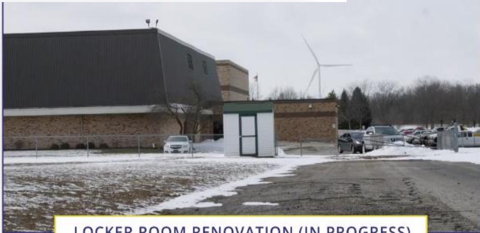
LOCKER ROOM RENOVATION (IN PROGRESS)
