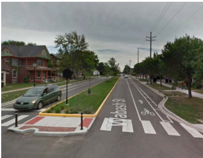
Bike lanes, green medians and native plantings were added during the Michigan City Wabash Street Improvements project.
