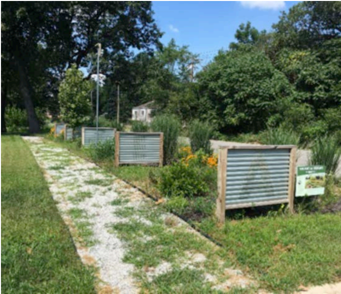
Gary's Aetna neighborhood incorporates public art into stormwater management.
