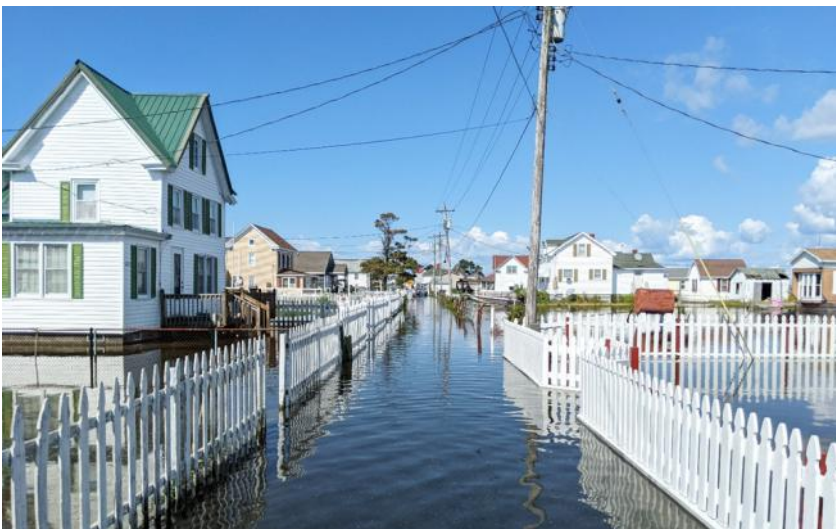
Main Ridge Road on Tangier Island during sunny-day flooding Photo: Lincoln L. Lewis, 20 September 2024
