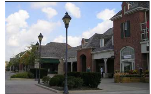
Pedestrian-scaled architecture in both urban (above) and suburban (below) settings.
