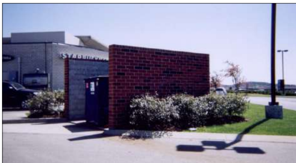
Figure 14 & 15: Screened Refuse Area
