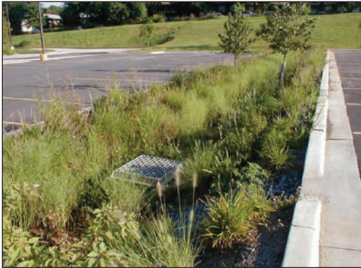
Example BMP: A swale situated between two rows of parking with curb indentations to allow natural water filtration
