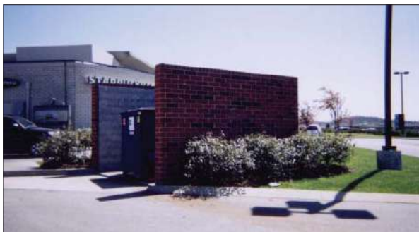
Figure 14 & 15: Screened Refuse Area
